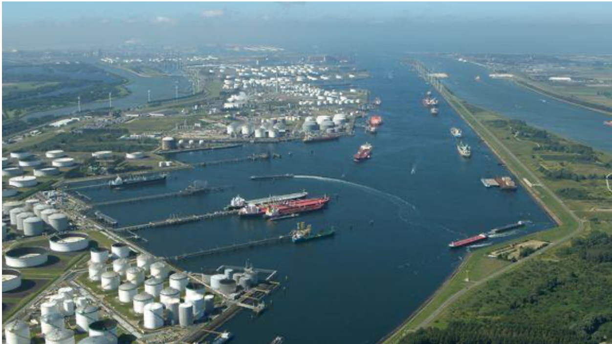
Figure 1. Showing the Port of Rotterdam with fuel storage tanks (in case of a future ammonia-fueled shipping, these tanks will store ammonia). https://www.portofrotterdam.com/en/news-and-press-releases/study-ammonia-cracker-realistic-and-safe-method-for-large-scale-hydrogen
