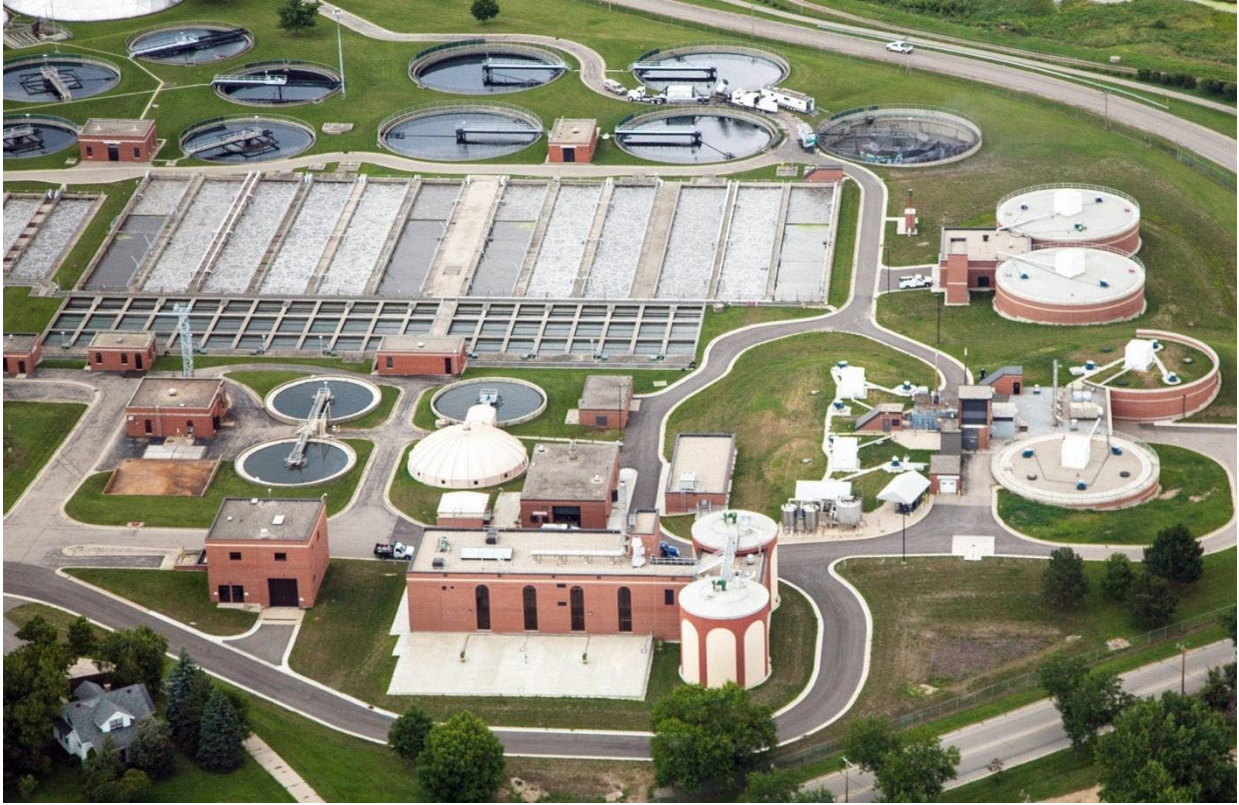
Figure 3: The Madison Metropolitan wastewater treatment facility showing different tanks used in the biological treatment stage.
