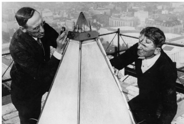
Two engineers inspecting the aluminum capstone on the Washington monument in 1934.
