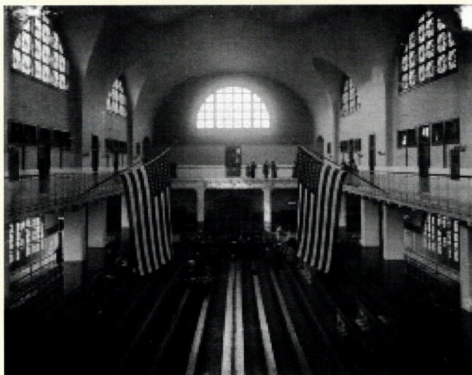
Inspection Room, Ellis Island, New York, NY. Early 20th century. Photo courtesy of the Library of Congress.
